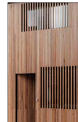
Facade R+1 : bardage bois vertical
